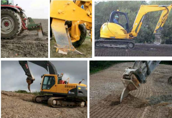
Figure 4-4: Top: (left to Right) Tractor-drawn tines; Large winged ripping tine; Topsoil rake on 3 tonne excavator. Bottom: Single ripper tooth for relieving compaction to a depth of 600mm
